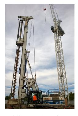
Frankipile engineers designed a secant pile wall basement retaining system with ground level propping off the capping beam which completely eliminated the need for ground anchors. This solution required careful coordination between the Main Contractor, the Engineer and Frankipile to ensure the design intent was achieved at the various stages of construction.
